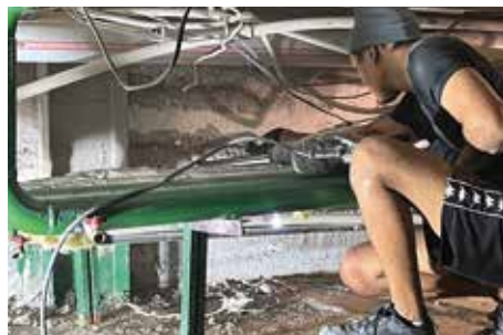
Barnabas-funded work making a church building in Kazakhstan resistant to flooding
