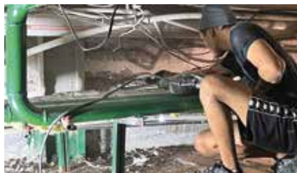
Barnabas-funded work making a church building in Kazakhstan resistant to flooding.
