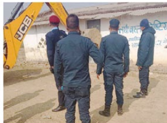
Police oversee the demolition of a church building in Nepalgunj, Nepal.
