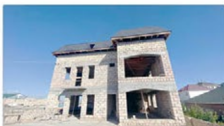
The multifunctional church building takes shape.
