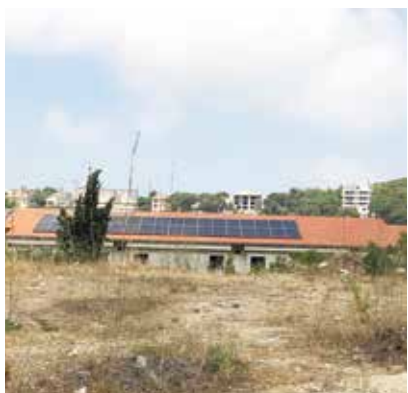
Barnabas-funded solar panels ensure a regular supply of electricity to this Christian elderly care home in Lebanon.
