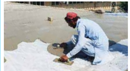
A workman resurfaces a section of the damaged hospital roof
