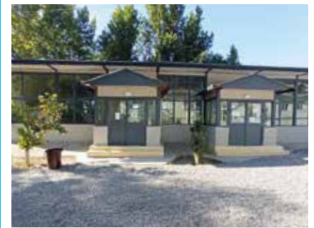
Church volunteers carried out much of the hall renovation themselves.
