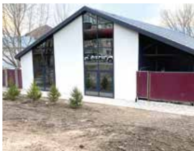
The newly repaired church in Kazakhstan.
