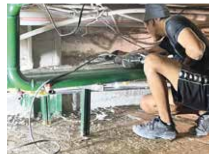
Barnabas-funded work underway on the church basement
