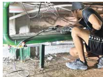
Barnabas-funded work underway on the church basement
