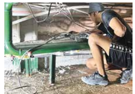
Barnabas-funded work underway on the church basement
