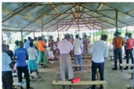
Christian refugees say they can now worship “without fear of rain, sunshine or wind” under the metal roof
