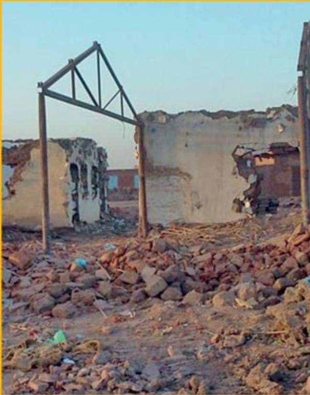
This church building was destroyed in Khartoum, capital of Sudan in 2013, when police stormed a gathering with bulldozers during a prayer vigil
